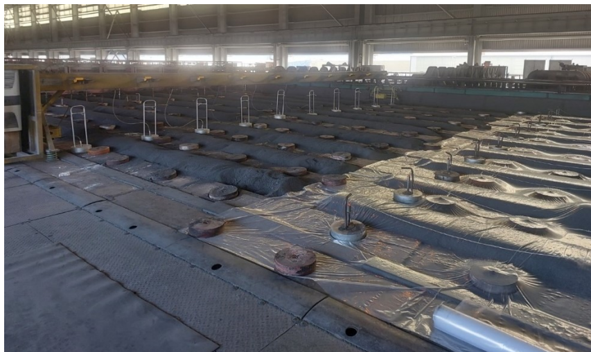
Figure 10. Use of plastic film in top of pre-heating zone.
